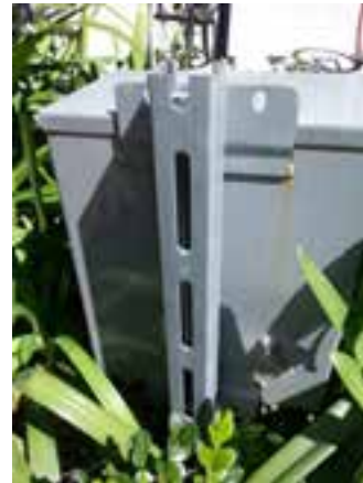
Enclosure on Unistrut in Planter
