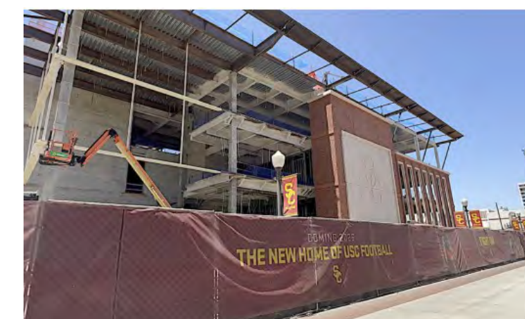
Bloom Football Performance Center Under Construction
