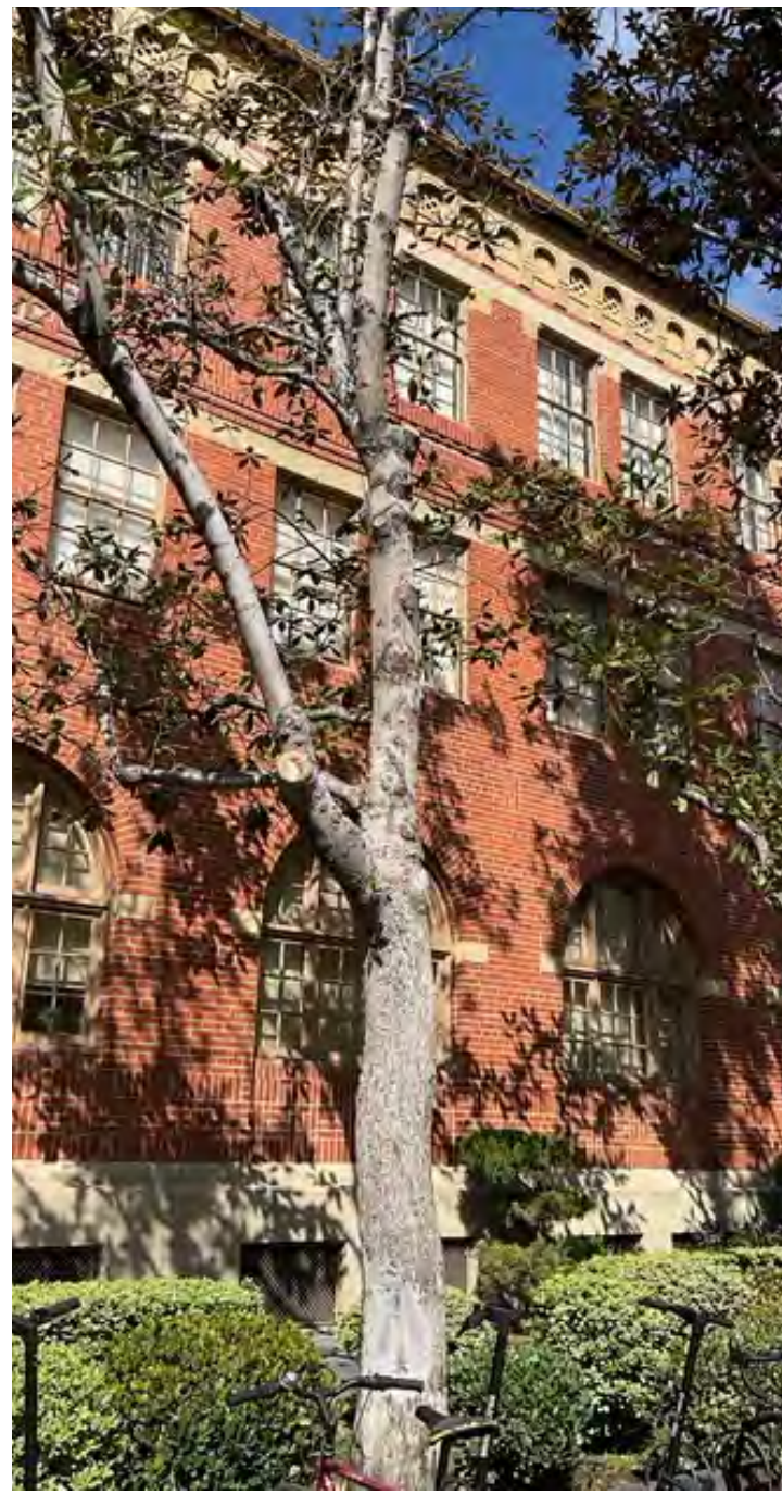
W09 Magnolia: To be Removed Within 5 Years Tree Decaying, With Weak Branches
